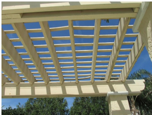
Warped wood at arbor
