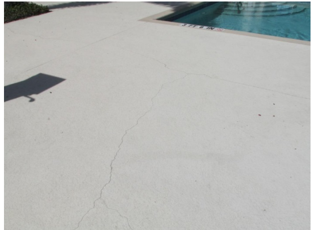
Note hairline cracks in deck
