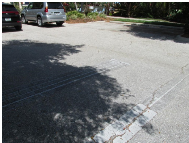
Note cracks at asphalt pavement parking area
