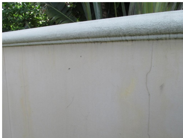
Perimeter wall with cracks noted
