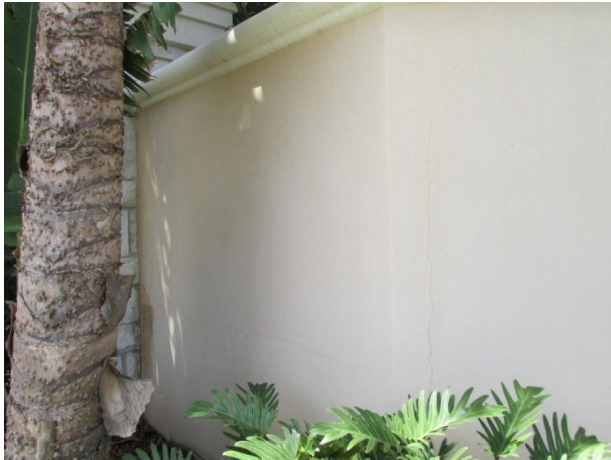
Perimeter wall with cracks noted
