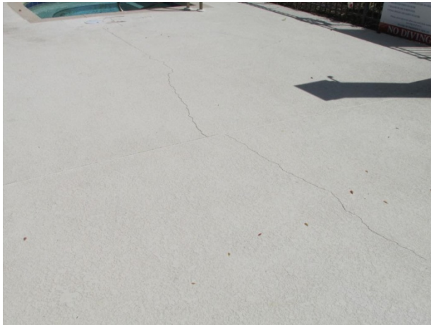
Note hairline cracks in deck
