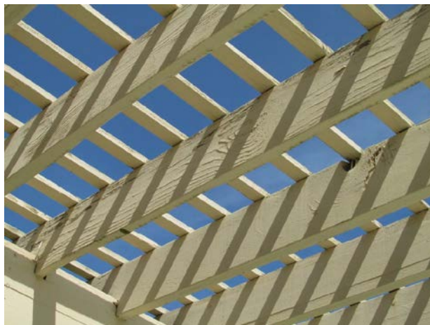
Peeling paint at wood arbor
